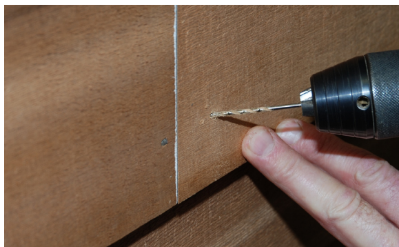
Figure 4—Pre-drill siding prior to nailing at the end of a piece of siding.
