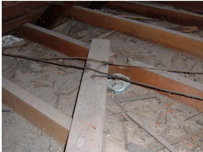
Fig. 2 – Knob-and-Tube Wiring From House OR-1
