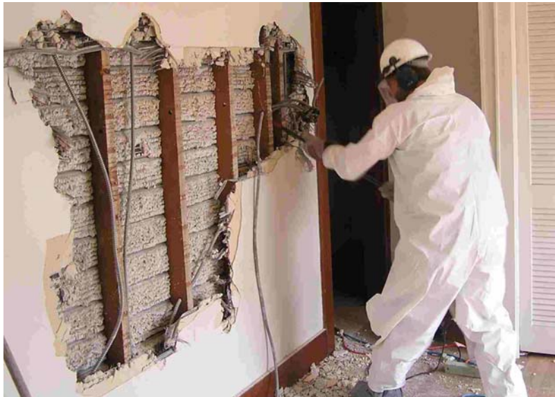
Fig 3 – Old Armored Cable Being Removed From House IL-1
