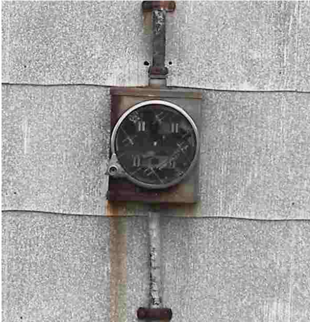
Fig. 10 – Meter Socket With Corrosion From House NY-1
