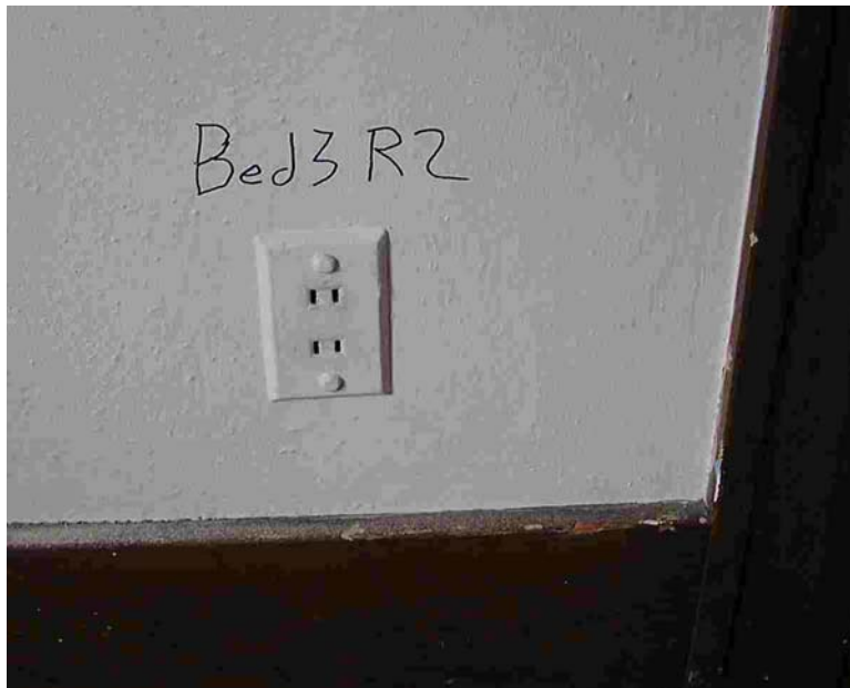
Fig. 18 – House IL-1 Receptacle From the 1920s
